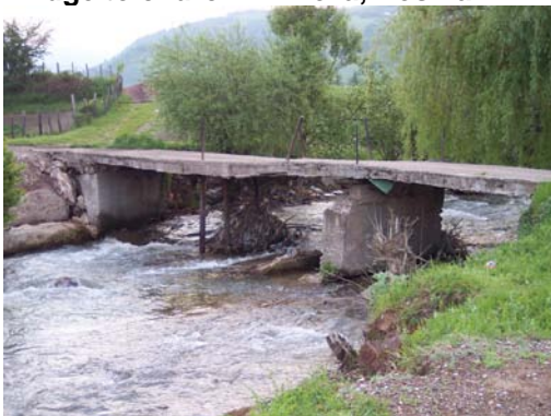
Bridge to church in Breza, Bosnia
